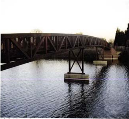
Indicative bridge style. Photos provided by Sarum Hardwood Structures
